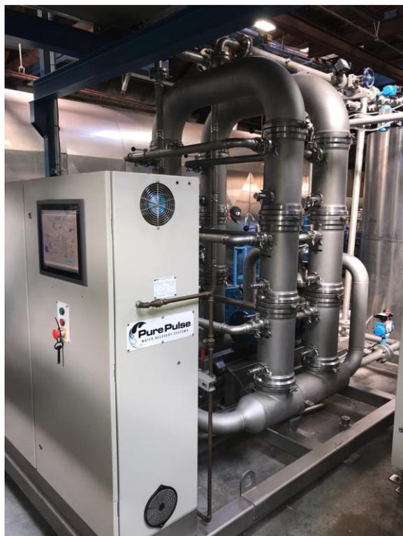
**Project description:** G2O Water Technologies Ltd., Hydrasyst Membranes UK Ltd. and Johnsons PLC propose to design and install a NanoPulse laundry filtration device at Johnson's industrial laundry site in Shaftesbury, UK. The NanoPulse system is an innovative solution for recycling waste water from the laundry sites, delivering energy savings by reducing the amount of heating required between wash cycles.
